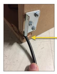
Chase power cord for Finish box out mouse hole at side of cabinet as shown.
